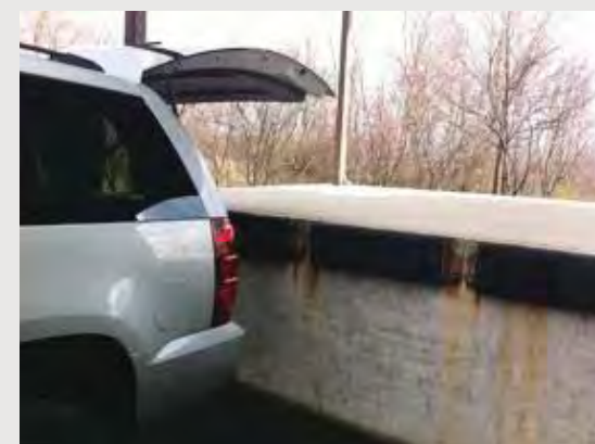
2. The building loading dock was constructed for tractor trailers – not for the types of vehicles used by AL researchers. Vehicle loading and unloading of equipment and gear for field research is difficult due to the configuration of the loading dock and its exposure to the elements.
