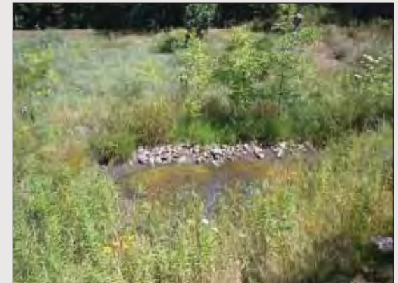
2. Stormwater Collection Pond
